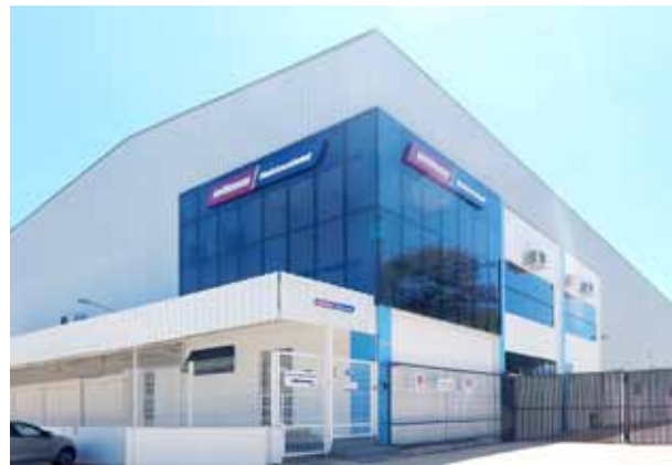
New building of WITTMANN BATTENFELD do Brasil.
