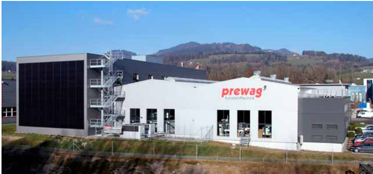
Prewag company site in Eschenbach-Neuhaus, Switzerland, viewed from the south. In this picture, the solar panels on the extension building constructed in 2016 can be recognized on the left.
