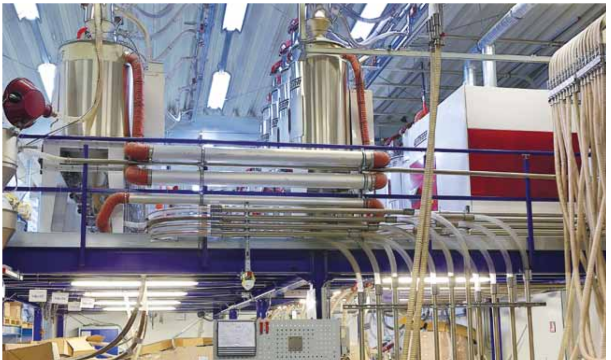
Views of the central WITTMANN material drying and conveying system at Pollmann in Karlstein, Lower Austria.
